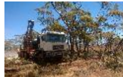
Drilling at Menninnie Dam
